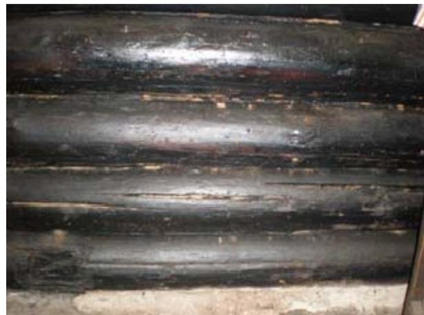
Figure 3. 5 Insect damage of wood.
