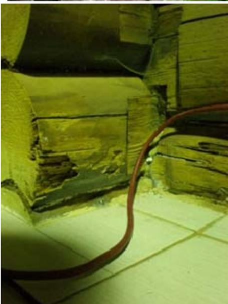
Figure 3. 1 Evidence of brown rot outside and inside of beams.
