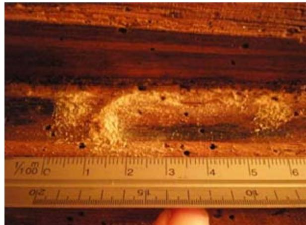
Figure 3. 6 Anobium damage in the wood.
