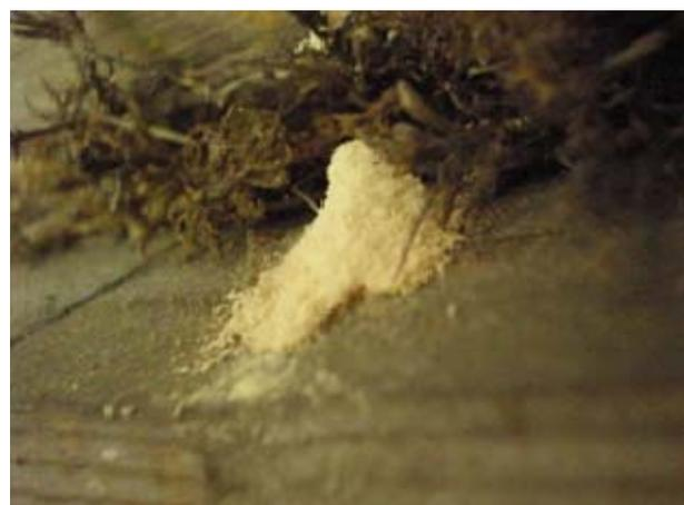
Figure 3. 7 Evidence of HYLOTRUPES BAJULUS attack.
