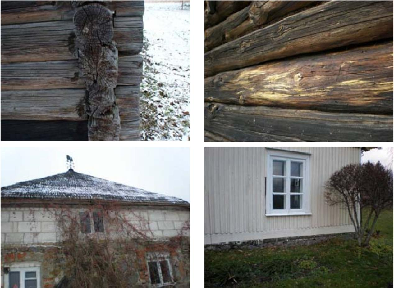
Figure 3. 9 Different kinds of problems causing damage which could lead finally to the moisture problems.
