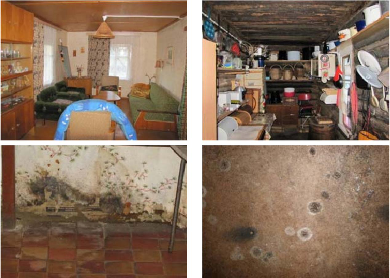
Figure 3. 4 Mould appearance on different materials.
