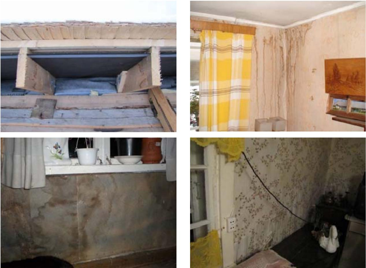
Figure 3. 8 Signs of moisture damage in buildings.
