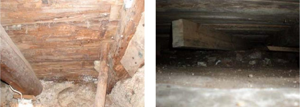
Figure 3. 2 White rot appearance in different constructional sites.
