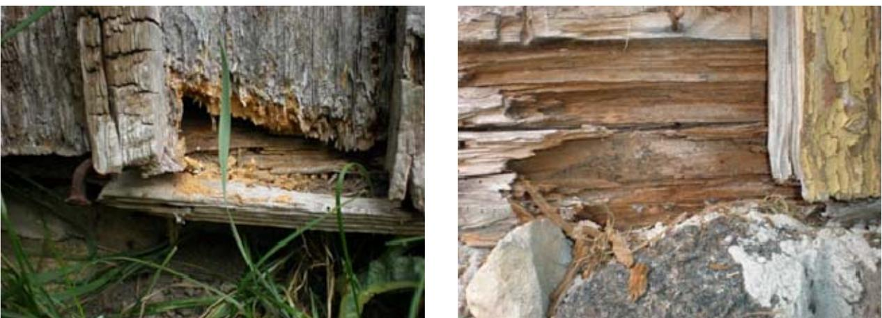
Figure 3. 3 Evidence of soft rot.
